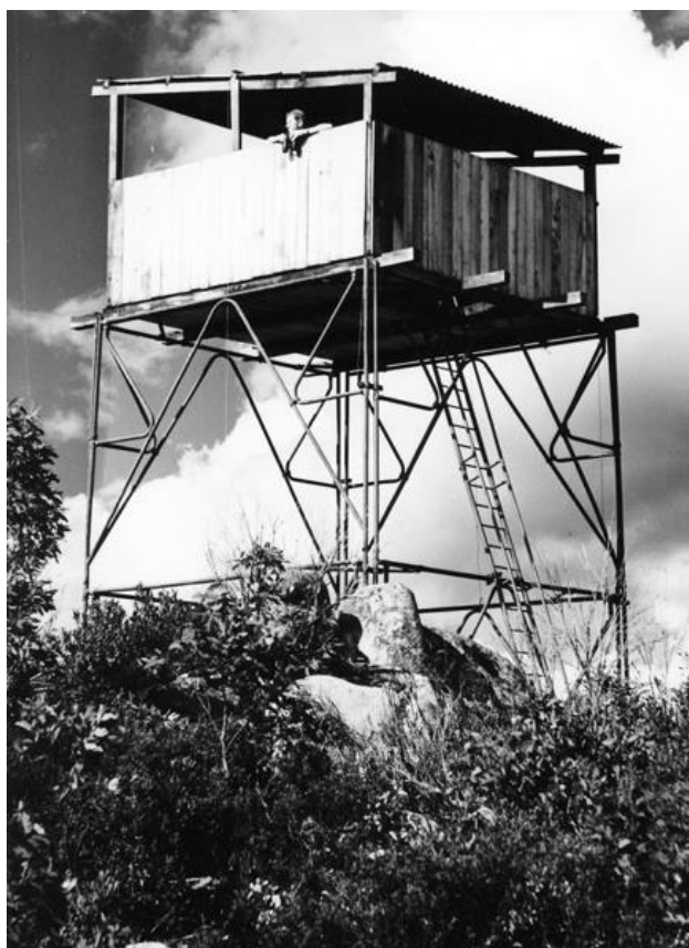
Mount Nugong, on the other hand, was built out of a metal-framed control tower scrounged from the RAAF base at Bairnsdale and erected over the summer of 1952-53. The legendary Bill Ah Chow spotted the Omeo #11 fire at Bindi from here. Photo FCRPA Collection.
