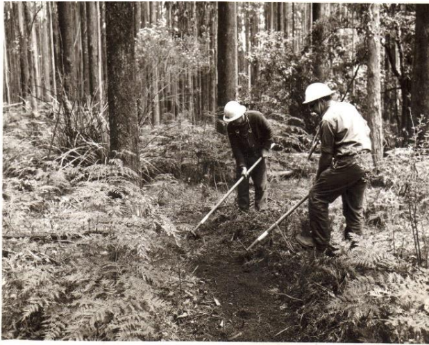
The first reference to the humble rakehoe was in the 1955-56 FCV annual report although it's more commonly believed they are a Victorian variation of the American McLeod Tool developed in 1905. The Pulaski Fire Tool had been trialled but never found favour with Australian firefighters. Source: FCRPA collection.
